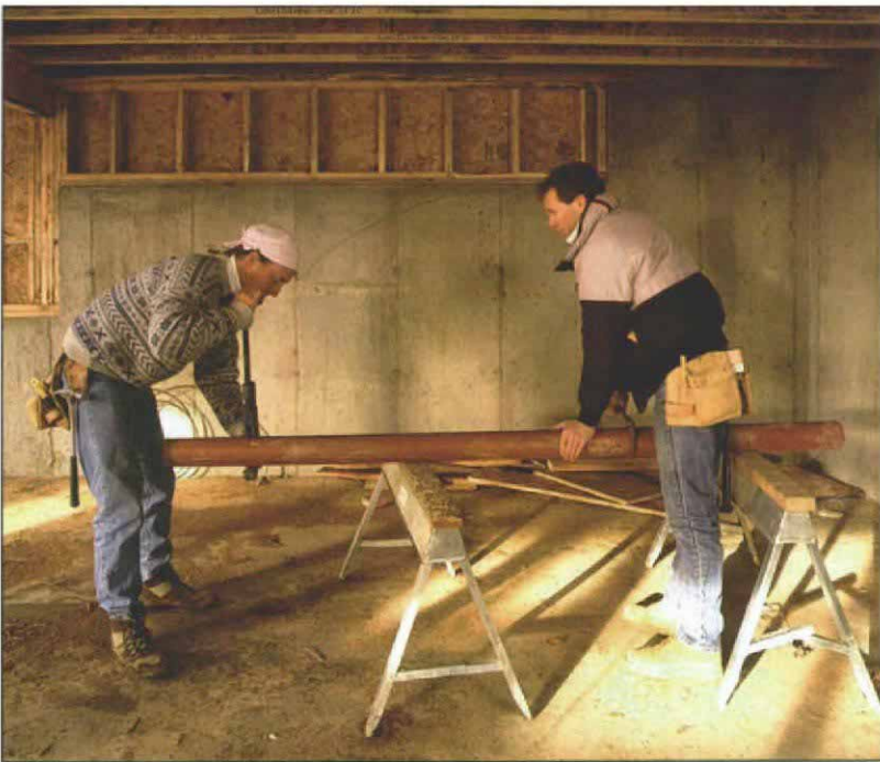
Cutting the column. Lally columns are steel tubes filled with concrete, and they're cut with a large pipe cutter. Once you cut through the pipe, knock off the end with a hammer, and chisel down any rough edges with a hammer claw.
